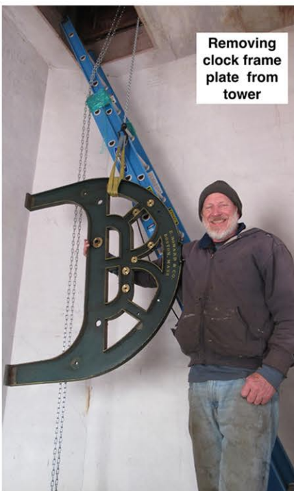
Mr. Graf lowers one of the clock frames out of the tower.
