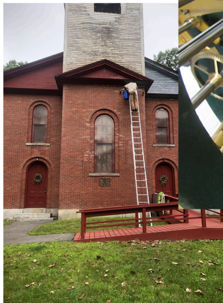
Re-painting the trim and wooden siding at front of the Meeting House. The clapboards of the clock tower will be replaced and painted red next year as the tower is restored.
