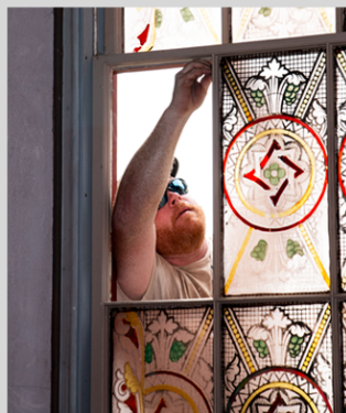
Andrew Moulton of Mid-Maine Restoration preps the wooden sash to receive a replacement pane of stenciled glass.
