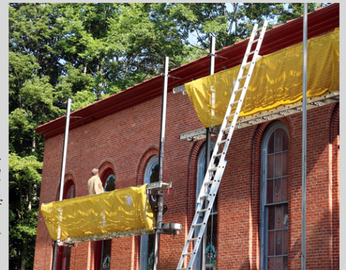
Andrew Moulton of Mid-Maine Restoration preps the wooden sash to receive a replacement pane of stenciled glass.
