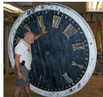
The clock faces were totally restored and re-gilded in 1985. By 2015 (only 30 years later) they were in ruinous condition. Now they require a complete overhaul before they can be re-installed. Rotted wood will have to be replaced, exterior molding reformed, new numbers made and 28.5 gold leaf used to make everything right.
